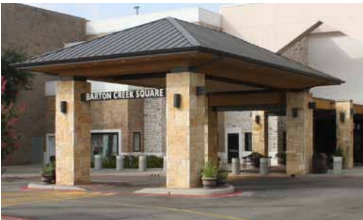
Barton Creek Square Mall - Austin, TX
